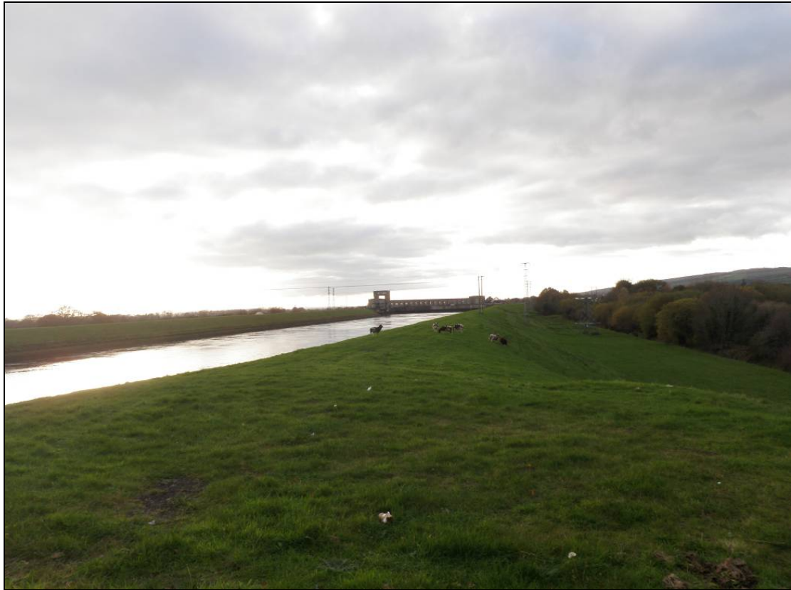
Photo 3.4.2 – Headrace Canal at Ardnacrusha
