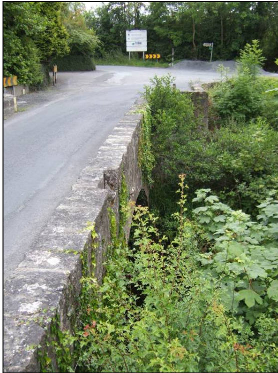
Plate 12 – BH 48 (bridge), facing south
