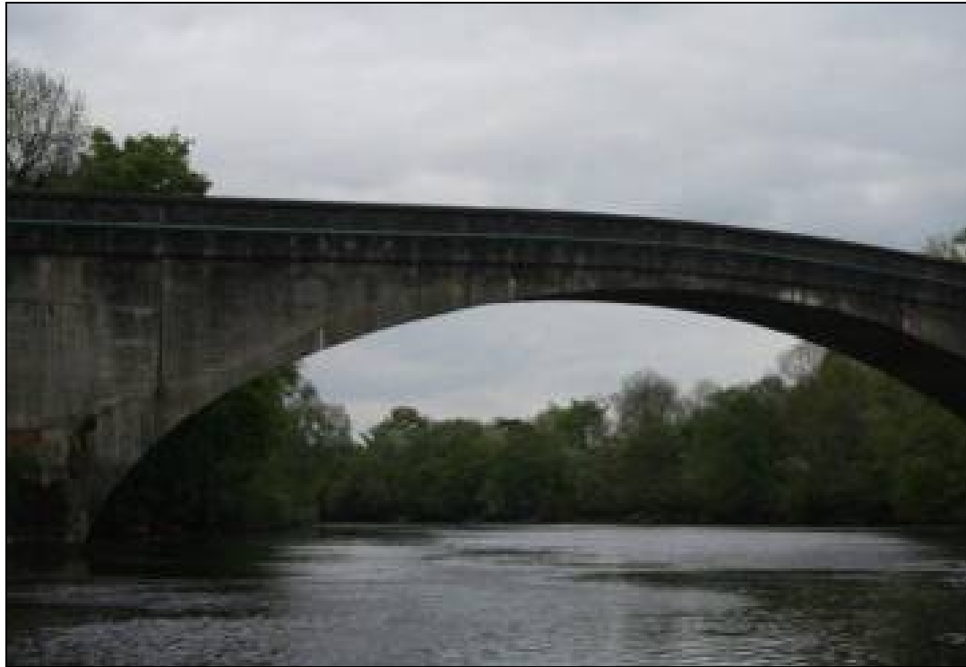
Photo 3.4.5 – Tailrace Canal Crossing, Parteen Bridge
