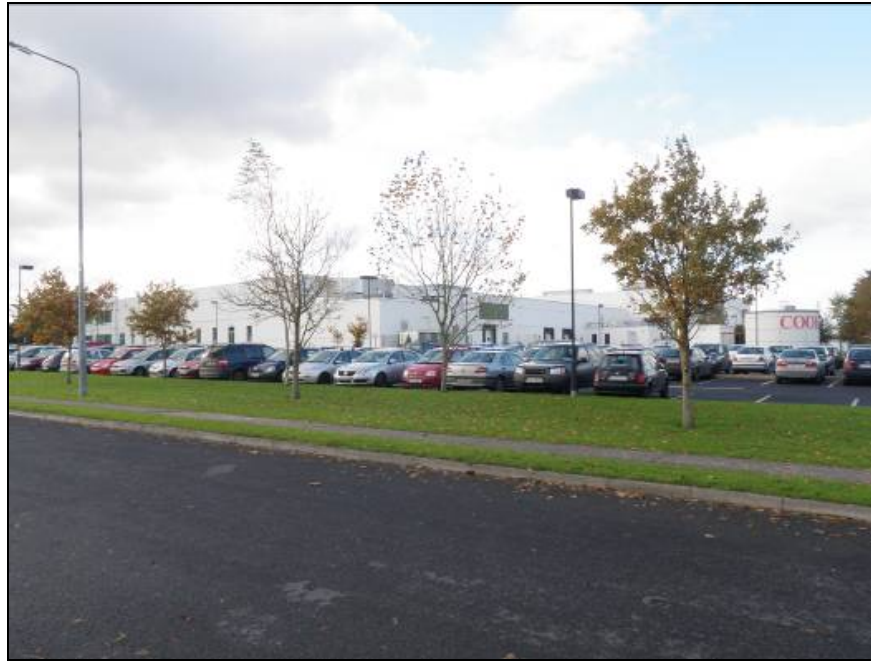
Photo 3.7.2 – COOK Ireland Facility
