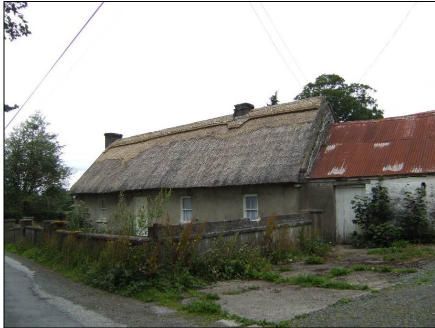
Plate 13 – BH 50 (vernacular cottage), facing northwest
