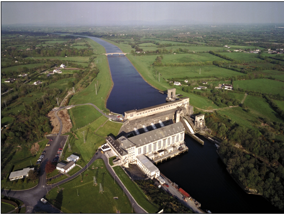
Plate 3.6.1 – Aerial View of Ardnacrusha Power Station
