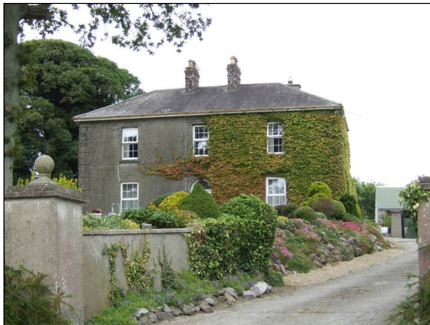
Plate 14 – BH 51 (large farm house), facing east northeast
