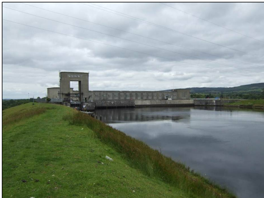
Plate 9 – BH 5 (Ardnacrusha Power Station), facing west
