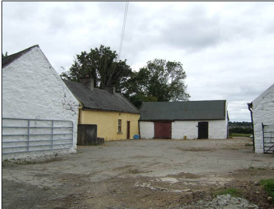
Plate 15 – BH 52 (vernacular farmyard), facing west
