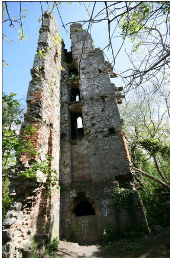
Plate 7 – AH 1/BH 26 (Plassy Mill ruins), facing south
