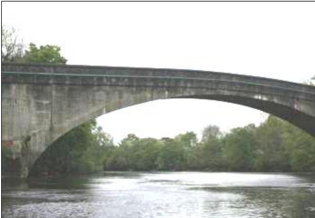
Photo 4.5 – Tailrace Canal Crossing, Parteen Bridge
