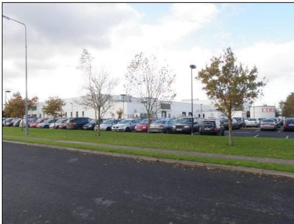
Photo 7.2 – COOK Ireland Facility
