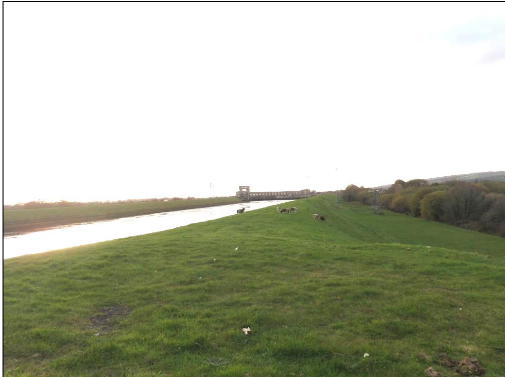
Photo 4.2 – Headrace Canal at Ardnacrusha
