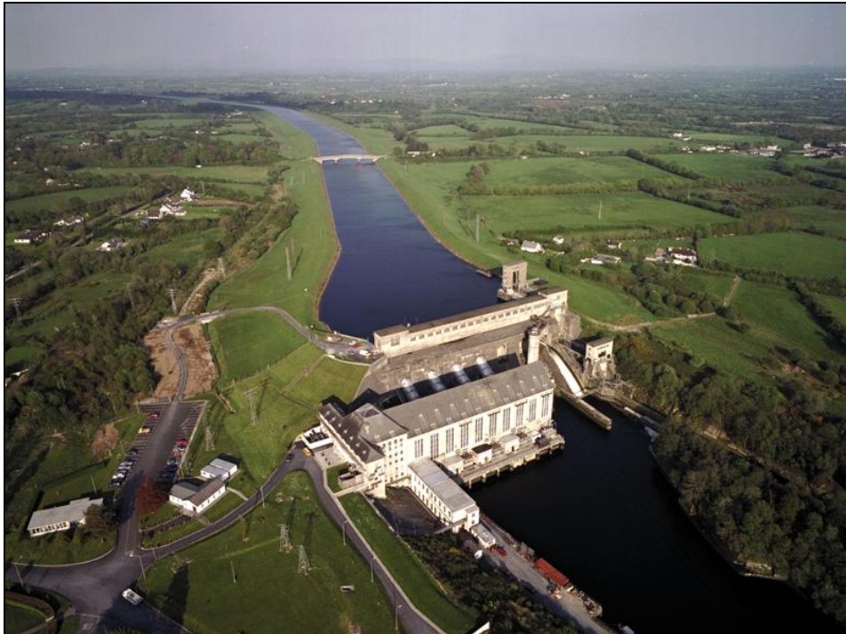
Plate 6.1 – Aerial View of Ardnacrusha Power Station
