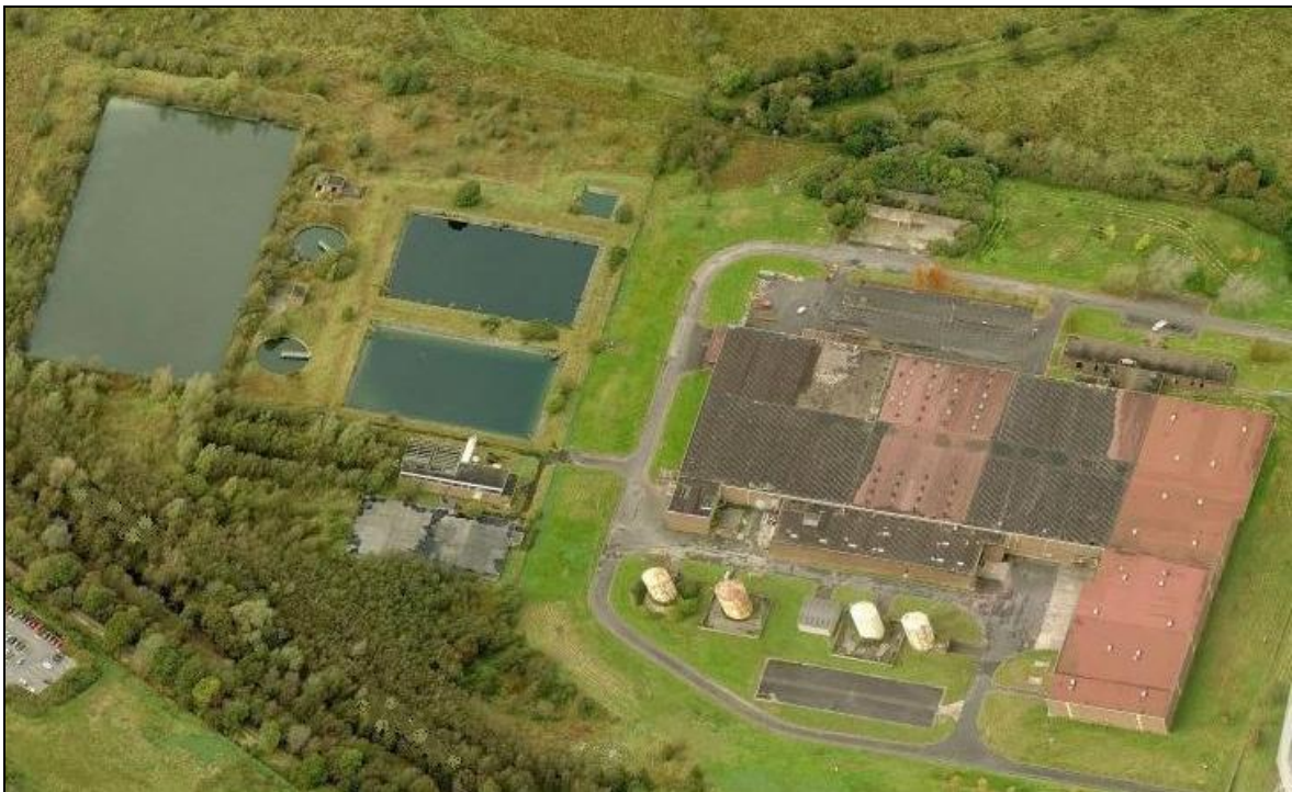
Plate 7.4 – Treatment Facilities, Gillogue
