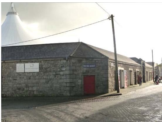
Existing Milk Market, refurbished recently
